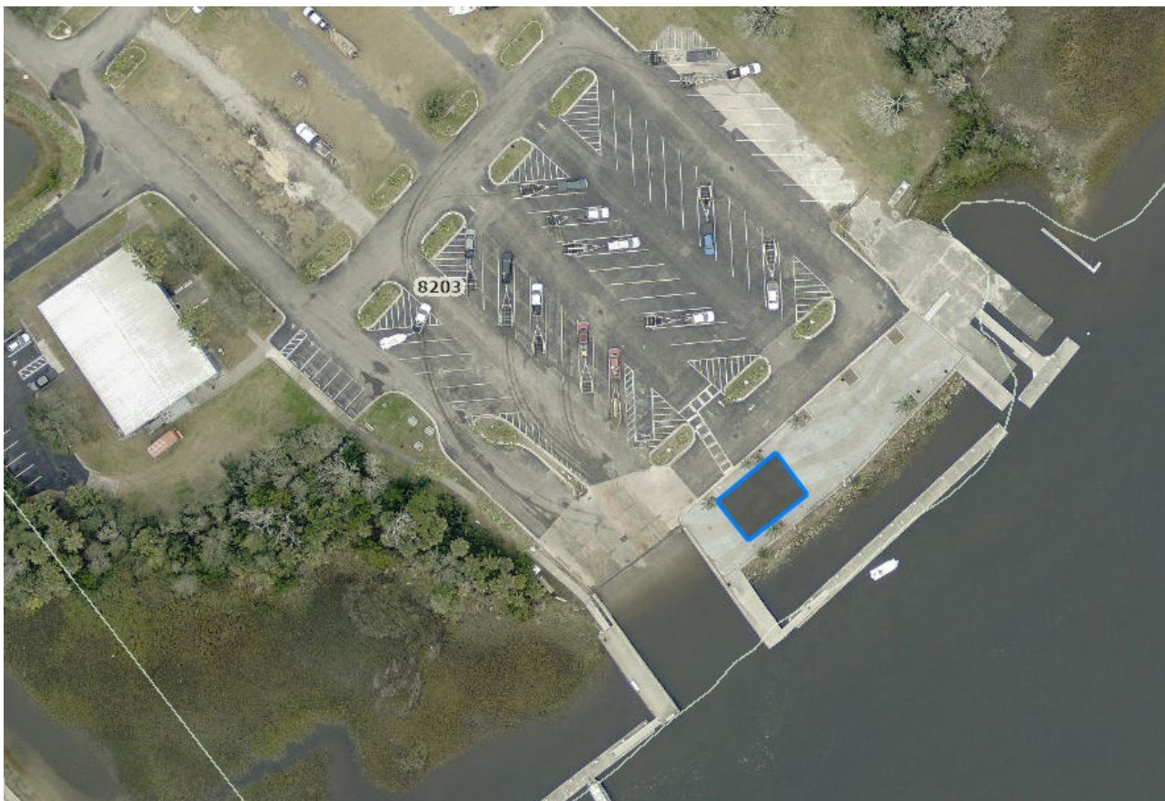
Sisters Creek Boat Ramp – events pavilion (design/build)
